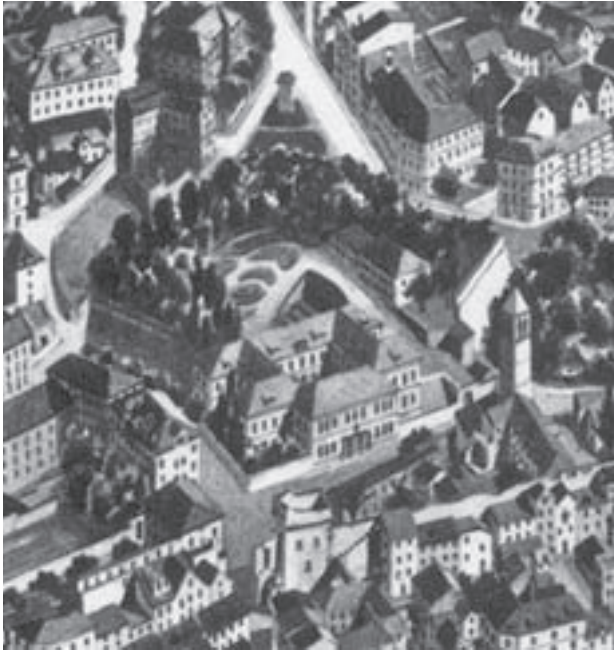
Slika 2. Stara gradska bolnica u Splitu Figure 2. Old city hospital in Split
